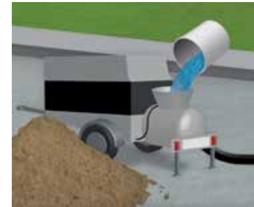
3 Adding the defined water quantity, caution - mix time!
