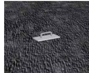
5 Compacting the screed mortar
