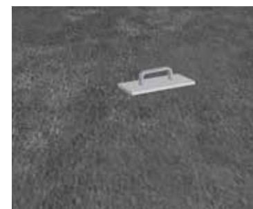
7 Rubbing up and finishing the screed surface
