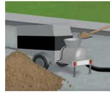
1 Filling the screed machine with aggregate
