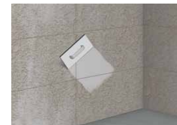
6 Sliding diagonally across excess joint mortar
