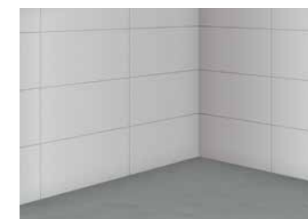
10 Finished and jointed wall surface
