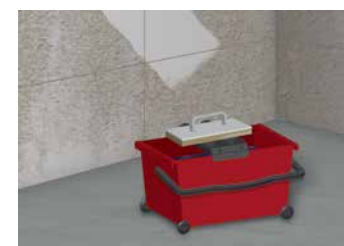
7 Moisten and press out the clean sponge board
