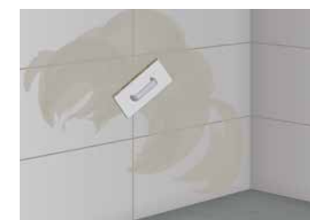
8 Emulsify the joint mortar after setting
