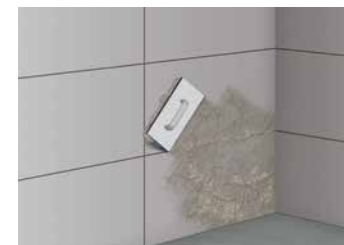
5 Apply the joint mortar
