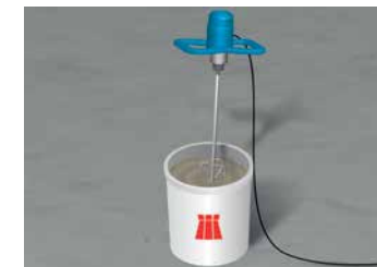
4 Mix the joint mortar
