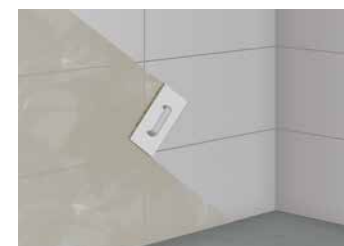
9 Rinsing off surfaces diagonally to the joint direction
