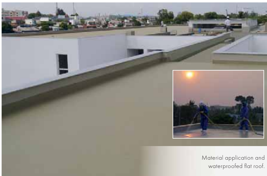
GEPOTECH® application demonstration on a flat roof in Vietnam.
