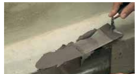
ASOCRET-M30 as a repair mortar.
