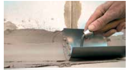
Forming a coved fillet with ASOCRET-M30.
