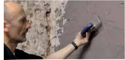
For smoothing or evening up from 3 mm thickness.
