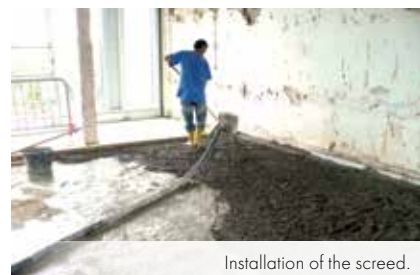
Installation of the screed.
