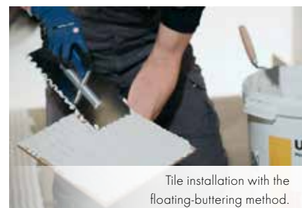
Combing out the tile adhesive.
