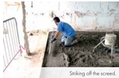
Installation of the screed.
