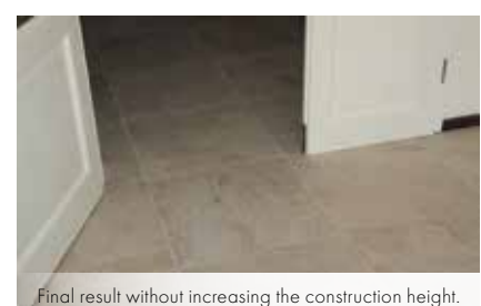
Final result without increasing the construction height.
