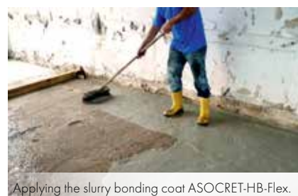
Applying the slurry bonding coat ASOCRET-HB-Flex.
