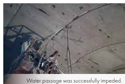
Polyurethane injection resin during application.
