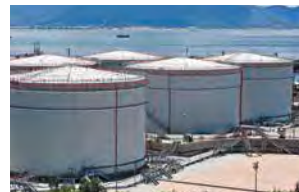
Tanks and containers
