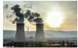
Power station cooling towers
