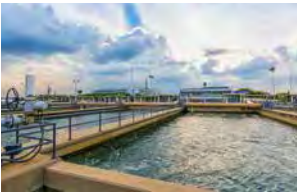
Collecting and retaining basins
