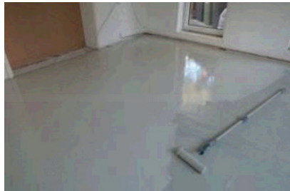
2. Application of sealing
