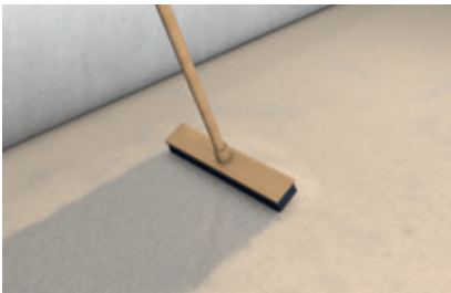
1. Clean priming, remove loose quartz sand
