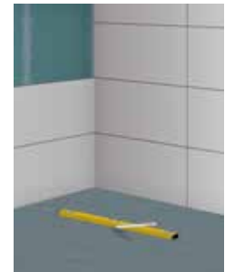
9 Setting out the floor
