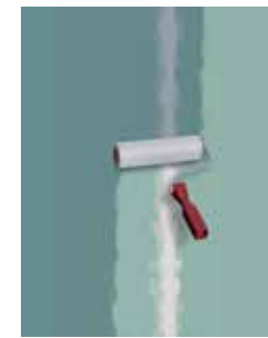
2 Priming the substrate, e.g. with ASO®-Unigrund
