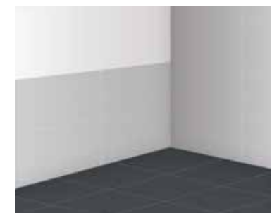
13 Finished area ready for use
