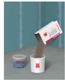
3 Adding the adhesive to a measuring bucket
