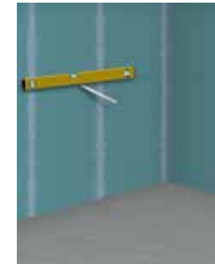
5 Setting out the wall
