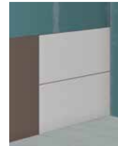
7 Fixing the wall tiles
