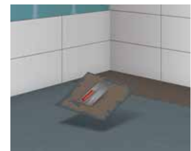
11 Applying a contact layer with large format tiles
