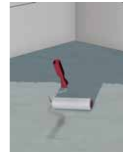
8 Priming the substrate, e.g. with ASO®-Unigrund
